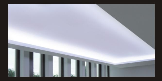
In modern architecture luminous ceilings and coved lighting have become discerning design features. They are the basis of a homogenous lighting design with a character similar to daylight. When implementing such lighting, it is important to prevent the characteristic dark zones in the gaps from one lamp to the next by overlapping the lamps.
